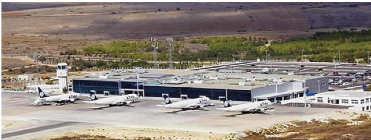
International Airport Lefkosa 1x 325 kVA
