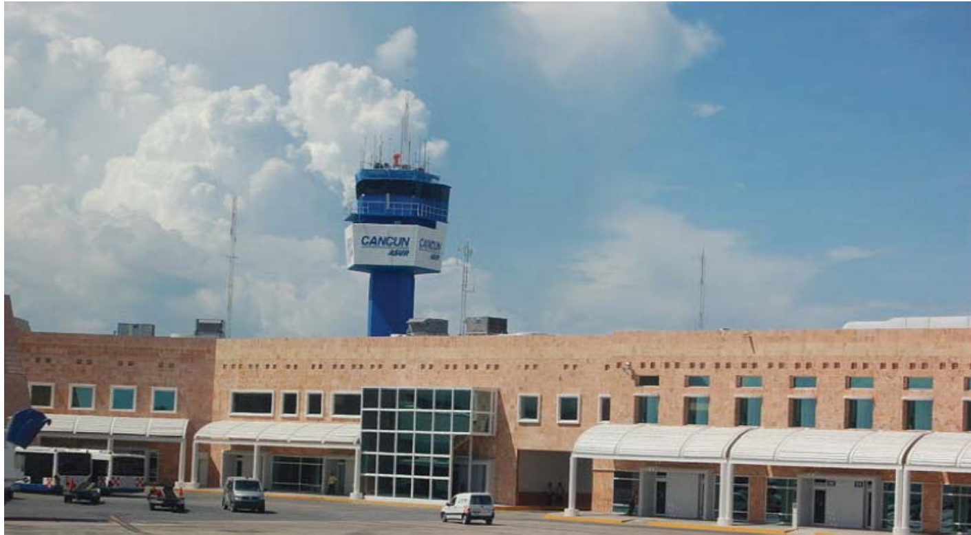
International Airport Cancun 1x 290 kVA
