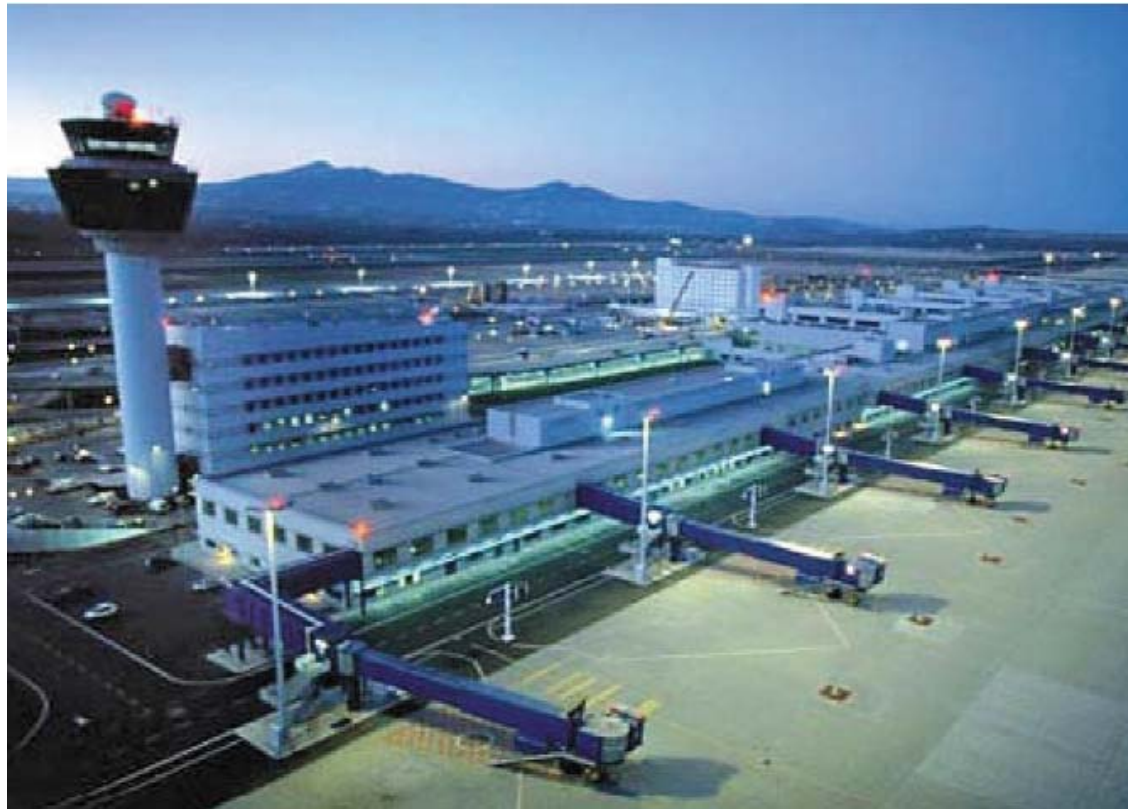
International Airport Athens: 4x 450 kVA
