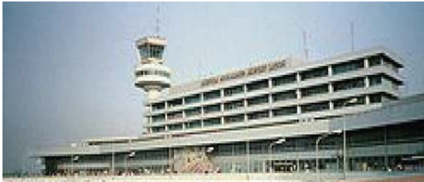
International Airport Lagos 2x 250 kVA
