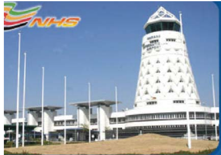
International Airports Harare and Bulawayo 2x 200 kVA 1x 50 kVA
